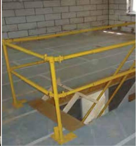
MKE Stairwell and edge protection guardrail system
