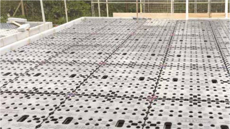
Swale deck safety decking / crash deck, 2m high x 1.2m<sup>2</sup> panels
