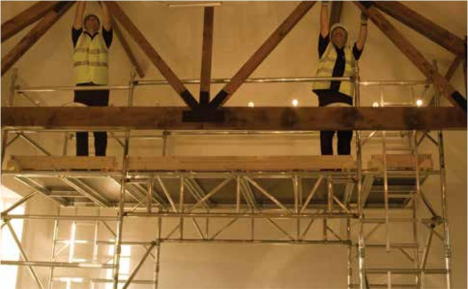
BoSS Tower Bridge Beams - 1.9m to 3.1m long, bridge beam kits for 1.8m or 2.5m long towers
