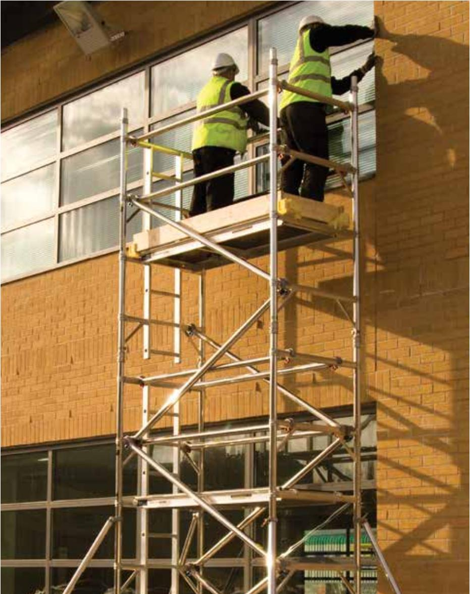
Platform lengths 1.8m, 2.5m and 3.2m. Platform heights ranging from 1.2m to 12.2m
